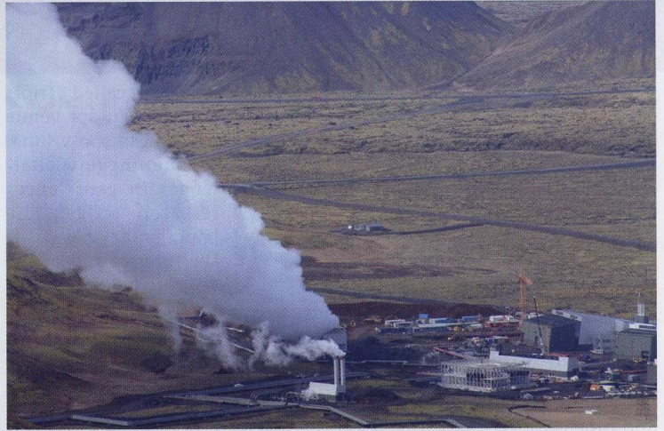
The CarbFix CO 2 injection site in southwest Iceland. The Hellisheidi power plant under construction is in the lower right, the moss-covered basaltic lava flow in the center of the figure, and the basaltic hyaloclastite (broken glass) mountains in the distance. The injection well is located in the lava fields in the upper left part of the photo. PHOTO: S. R. GÍSLASON
